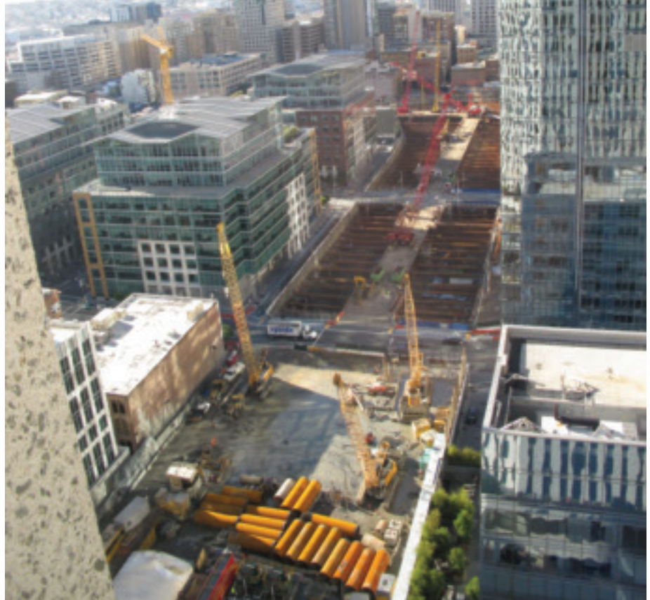
The huge Transbay Transit Center jobsite, in the heart of San Francisco, is four blocks long. At bottom are some of the 286 7-foot-diameter casings to be driven 240 feet down to hit bedrock.
