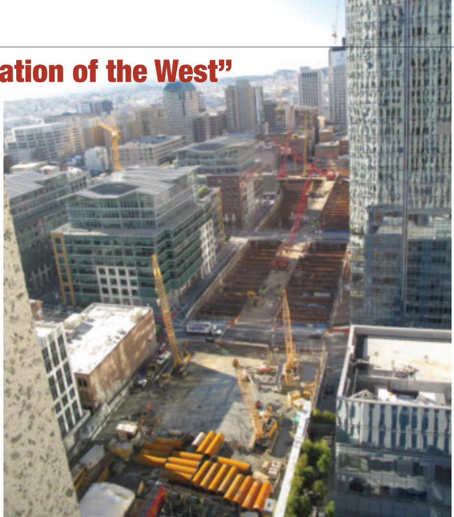
The huge Transbay Transit Center jobsite, in the heart of San Francisco, is four blocks long. At bottom are some of the 286 7-foot-diameter casings to be driven 240 feet down to hit bedrock.
